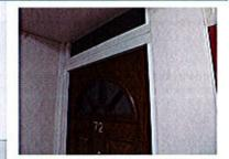
Recommendation: El 30 (30-minutes integrity and insulation) fire resisting glazing (and associated glazing channel and beading) should be installed in the fanlight(s) to flat entrance door(s) as noted. Fanlights above flats 12, 21, 24, 25, 29, 44, 45, 51 and 71 entrance doors
